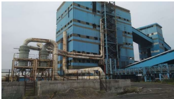
Fig 7: Dust extraction sytem at Coal crusher house
