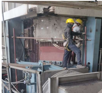
Fig 4: \text{NO}_x reduction – combustion modification works in boiler
