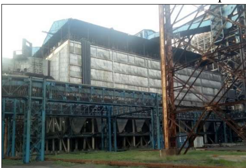
Fig 2: Electro Static Precipitator at NTECL
